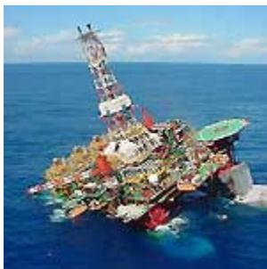
**Water flooded the platform's pontoons, causing the platform to list at a 25° angle.**
