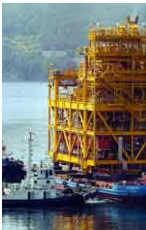
**Dalia FPSO has a water injection capacity of 405,000bpd, water treatment capacity of 265,000bpd and gas compression capacity of 8MMscf/d.**
