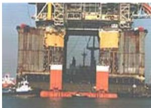
Kizomba A extended leg TLP showing the side leg supports. © Gerben van den Bosch.
