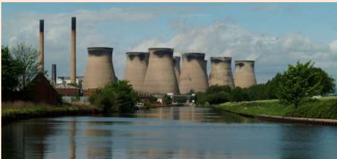
Ferrybridge Power Station image, courtesy of Scottish and Southern Energy
